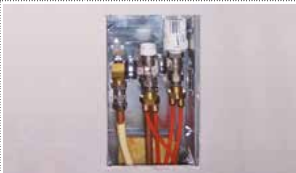
Control box option 2 with sub-manifold 2-port.
