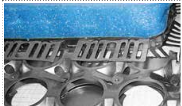
4 Insert brackets (HK) into border insulation tapes (minimum 3 pieces / m).
