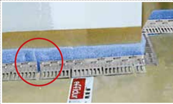
1 Simple forming of corners with border insulation tape. Overlapping of PE-foam.
