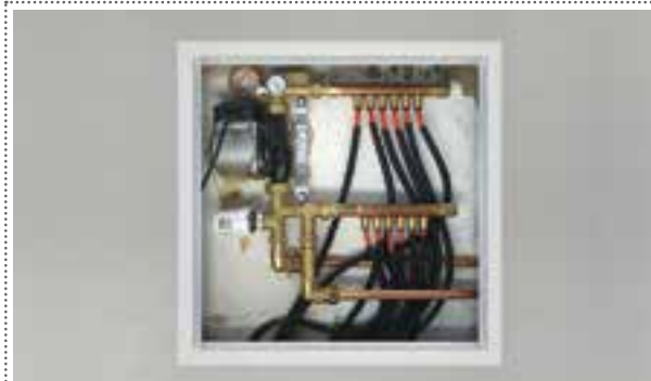
Manifold unit 6-port at control unit.
