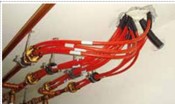
Zonal sub-distribution through the ceiling.
