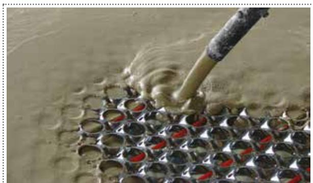
**2** Complete backfilling of the comb panels with system screed SFM.
